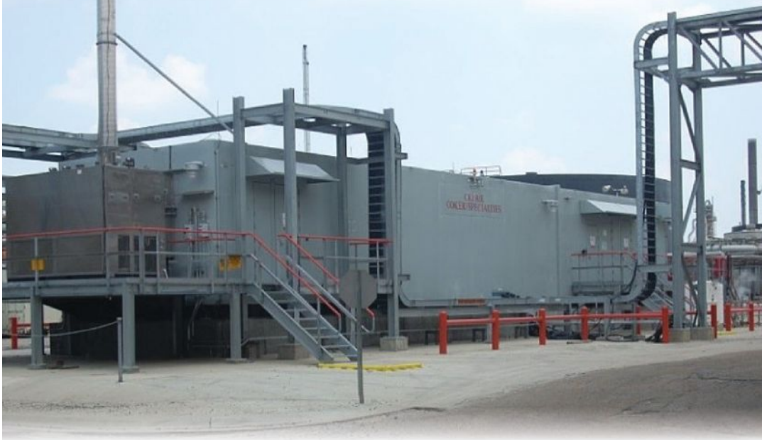
For a Gulf Coast refinery controls upgrade, Burrow Global designed remote instrument enclosures (RIEs) to house process control equipment and included redundant uninterruptible power supply (UPS) and HVAC systems. Courtesy: Burrow Global
